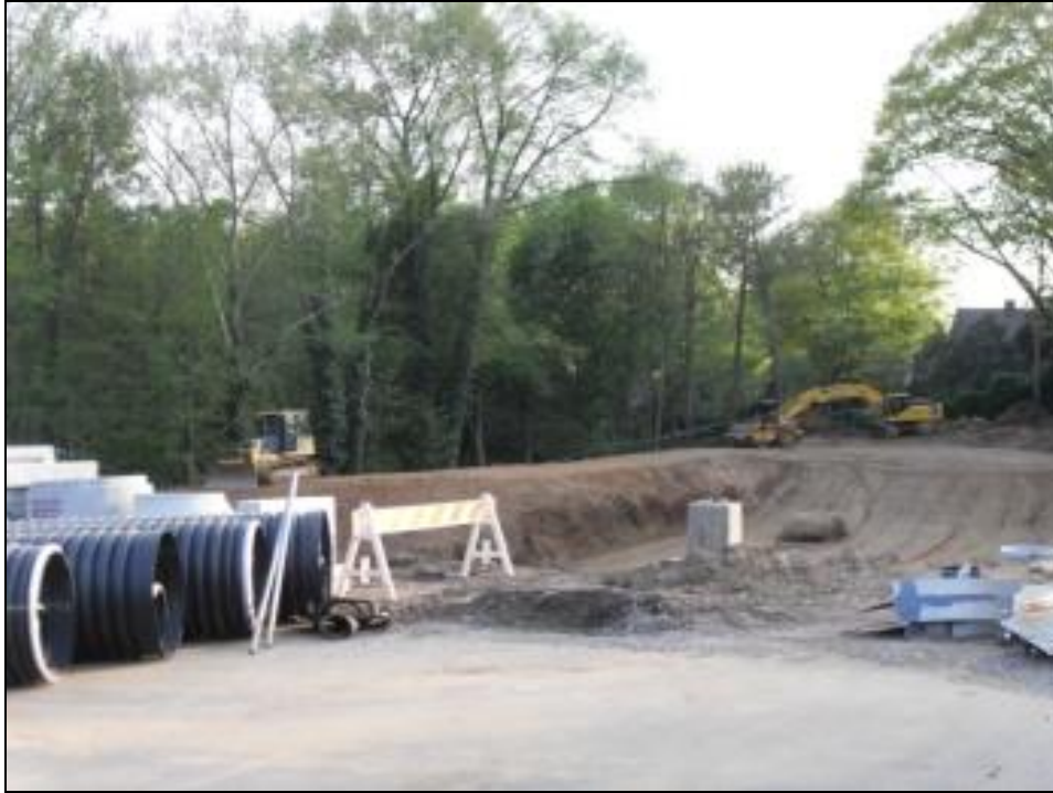
Figure 22. Photograph of the Springfield Square Shopping Center construction site.
