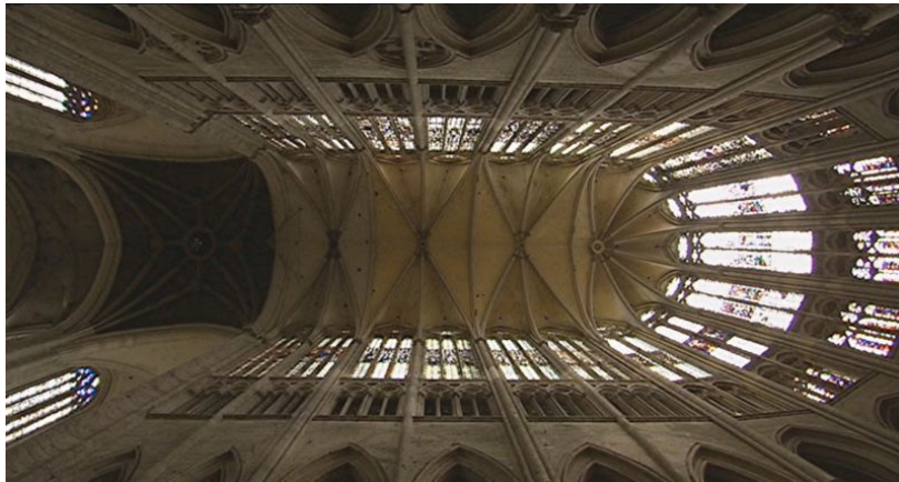
Figure 3: Ribbed sexpartite vault (six-part) in Beauvais Cathedral
