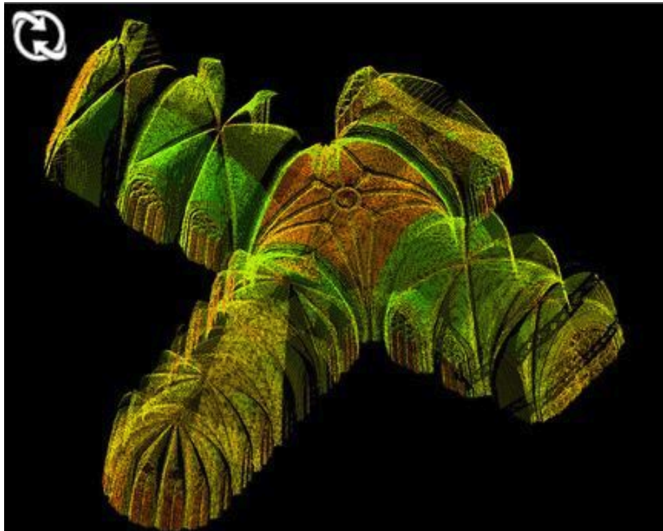
Figure 7: Beauvais choir vaults point cloud laser scan data from CyArk, demonstrating equilateral arch geometries used for modeling ideal quadripartite model.
